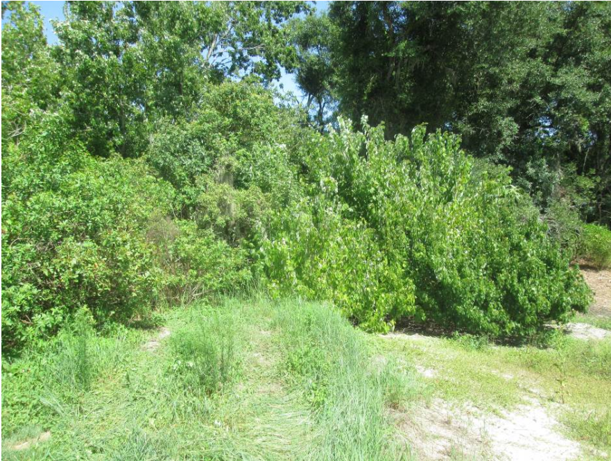
Item 5 - Pond 44 – Remove tree covering outfall weir
