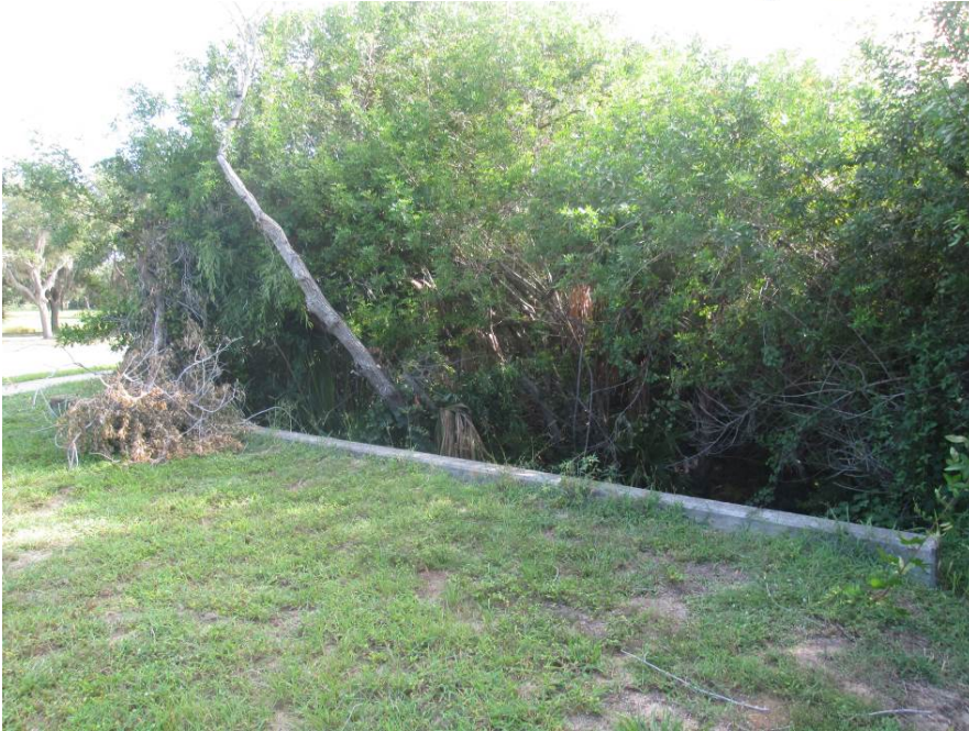
Item 18-Wingspan @ Pond 9–Remove broken tree branch, west headwall
