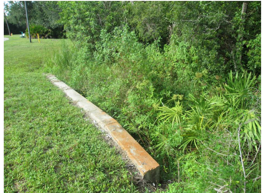
Item 14-Wingspan Way, n/o of Tara Preserve – Cut 15' veg. at east headwall
