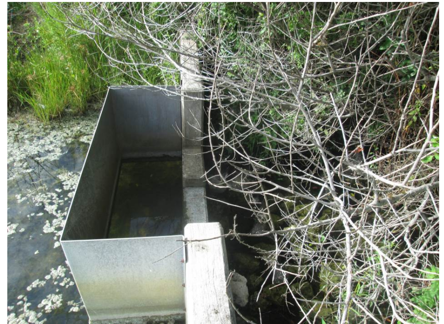
Item 17 - Pond 1 – Cut vegetation 15' behind weir
