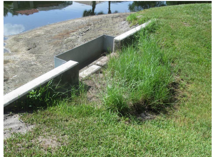
Item 4 -Pond 42 – Cut weeds behind weir
