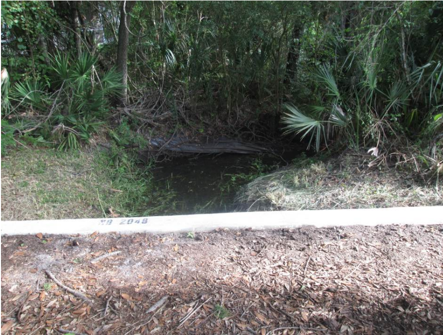
Item 16 - Wingspan at Covey Ct. – Remove silt fence south of headwall
