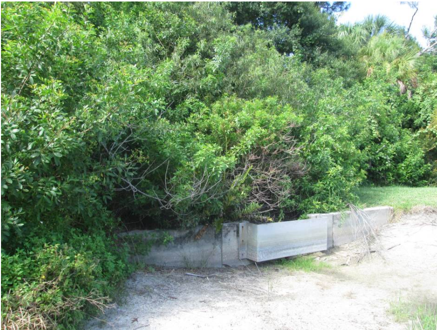
Item 8 - Pond 32 – Cut back vegetation 10' behind weir
