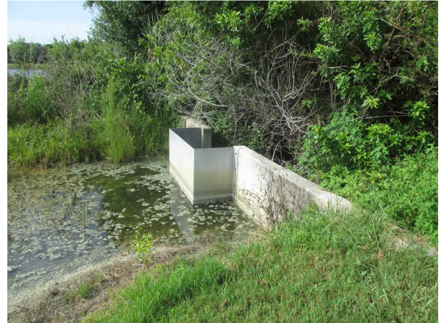
Item 17 - Pond 1 – Cut vegetation 15' behind weir
