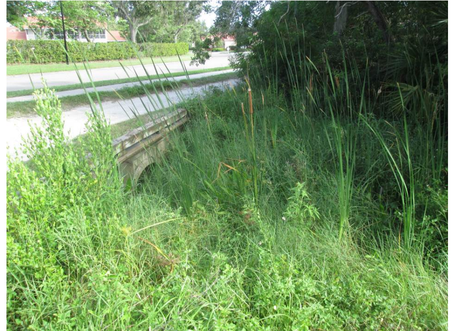
Item 14-Wingspan Way, n/o of Tara Preserve – Cut 15' veg at west headwall
